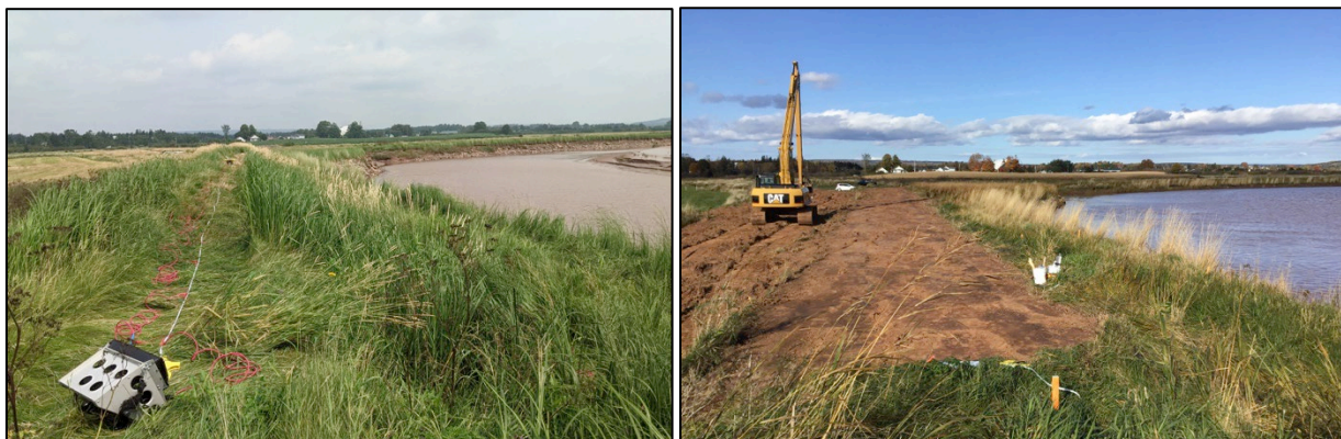
Agricultural dyke during resistivity surveying (left), and during breaching (right), 2021 field season.
