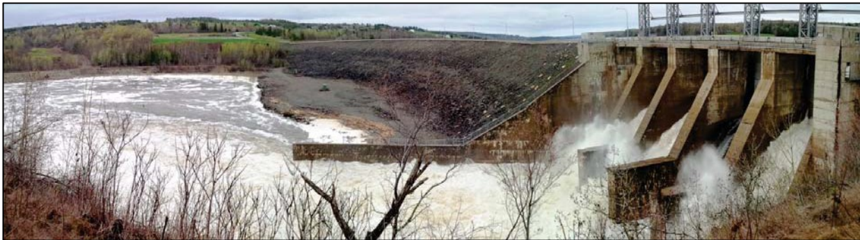
Embankment dam and diversion sluiceway at Mactaquac Generating Station during the spring freshet.
